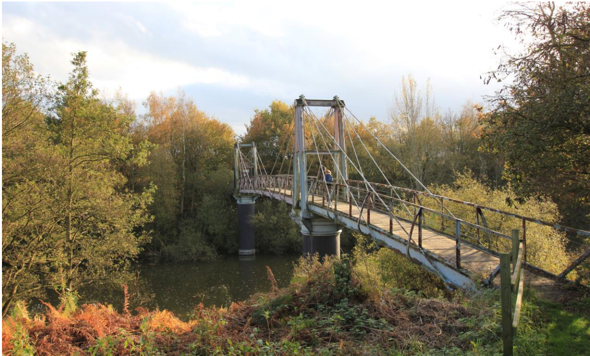
Footbridge on to No.3 bed
